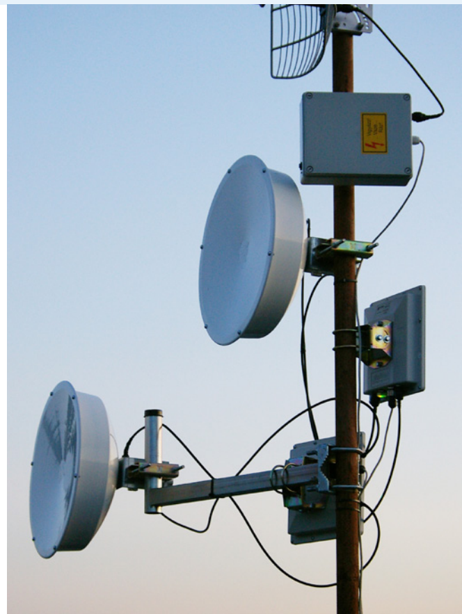
[ Figure 8 Cameroon long range link, with hop over Cameroon Mountain where solar power was used to supply electricity ]
