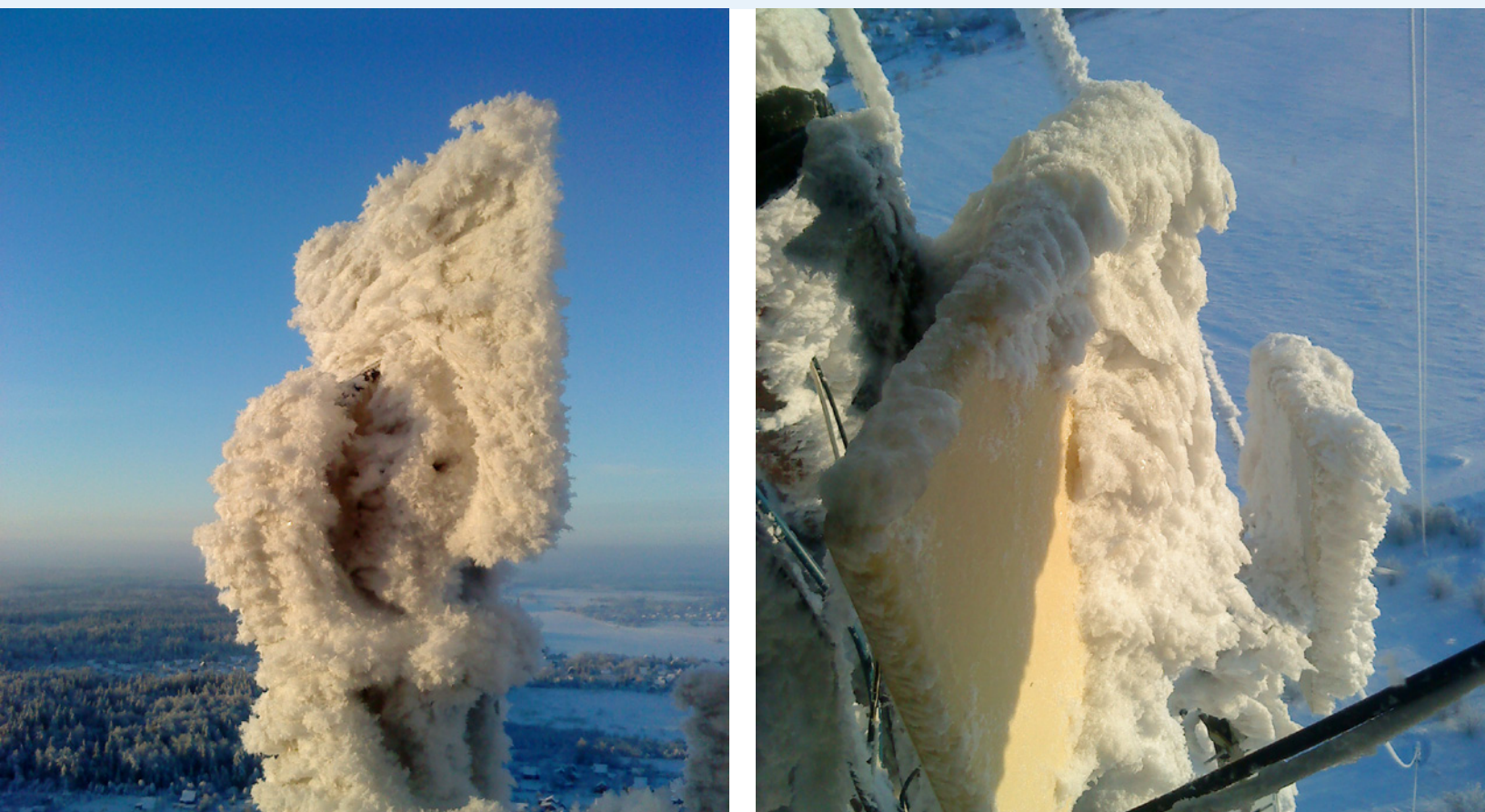
[ Figure 2 InfiNet wireless units in very low temperatures ]
